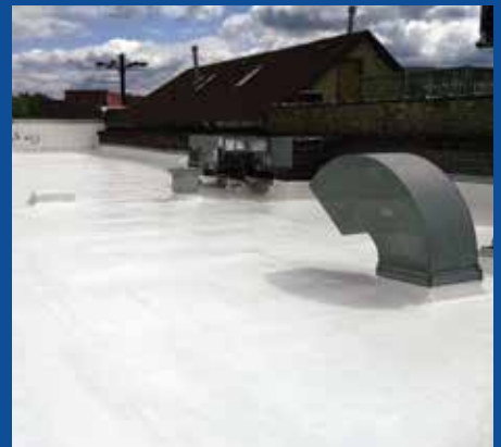
Liquid-Applied Roofing
