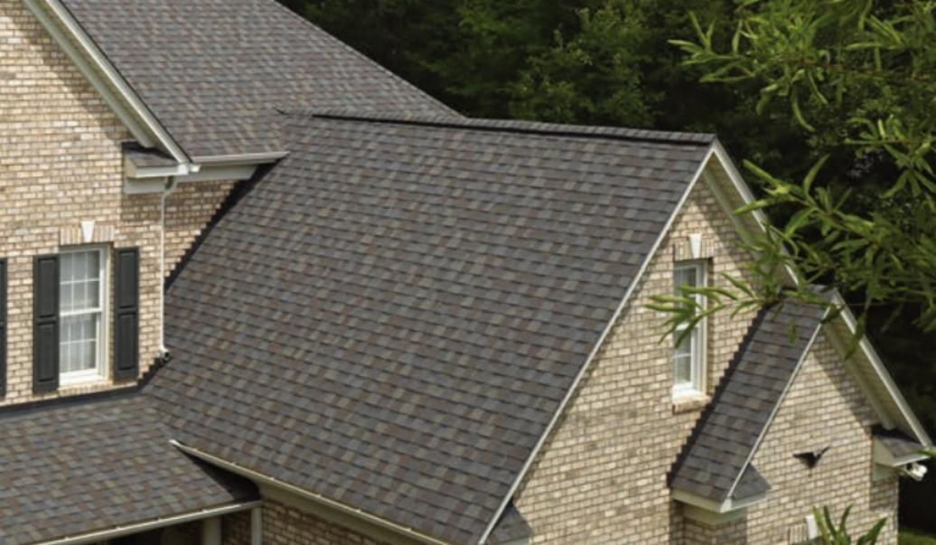
Since the early 1900s, the three-tab or strip shingle was the standard composition shingle installed on single family residences. Color was about the only appearance differentiation in this class of shingle.
